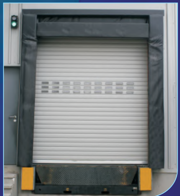
Dock Leveller Installation
